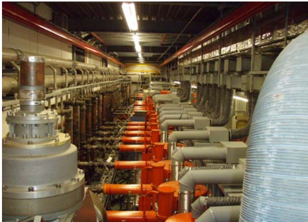
Figure 6: RF 108 MHz amplifier gallery.
