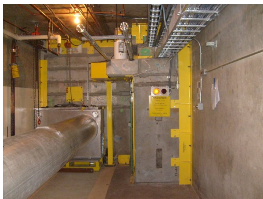
Figure 3: Completed shielding wall as seen from the tunnel in Sector 20.
