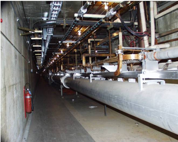
Figure 5: Sector 20 before the accelerator systems were removed. The linac is visible above the much larger alignment light pipe.
