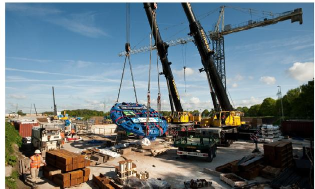
Figure 2: Arrival of the cutter head of the tunnel boring machine.
