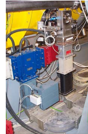
400kW circulator and 3 stub tuner in one of branch of ACC1 waveguide distribution
