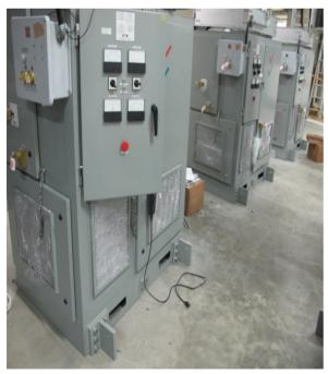
Figure 3: TPS quadruple magnet power converters.
