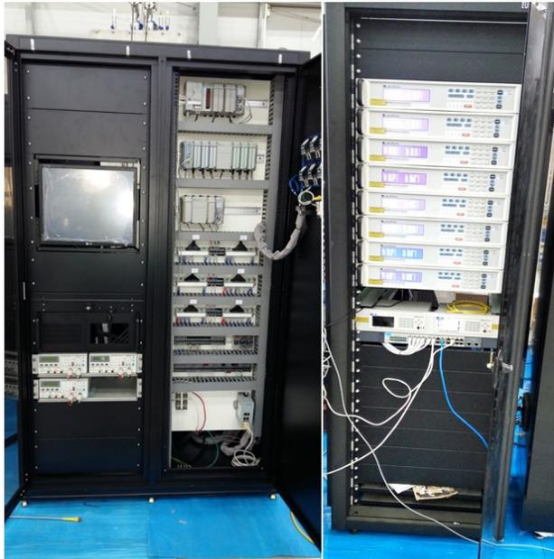
Figure 3: PLC rack and temperature monitors.
