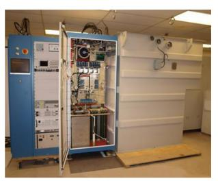
Figure 1: System designed for Oak Ridge National Laboratory Spallation Neutron Source. Design is optimized for long pulse operation with highest possible reliability and availabilityrequired for particle accelerator user facilities and test stands. High voltage cables connect to dummy load or klystrons not shown in figure.
