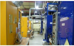
Figure 2: Three 300kW klystrons and KSUs.
