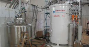
Figure 3: Helium cryoplant during commissioning phase.
