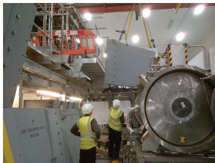
Figure 6: Installation of the MICE PRY south side in the MICE hall.
