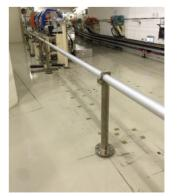
Figure 3: The support of isolation tube are adjusted and positioned on the exact location of ground in the straight section of TPS storage ring.
