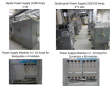
Figure 1: Large and small power supplies for the dipole, quadrupole, sextupole and correctors of TPS booster synchrotron respectively.
