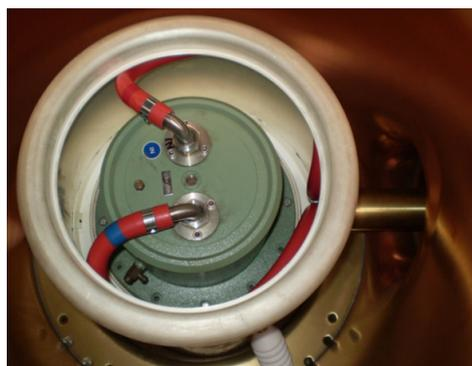
Figure 1: TH116 Triode installed in HT tank.
