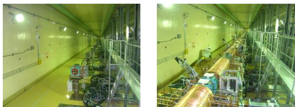
Figure 1: Linac tunnel before (left) and after (right) the installation of the ACS linac.
