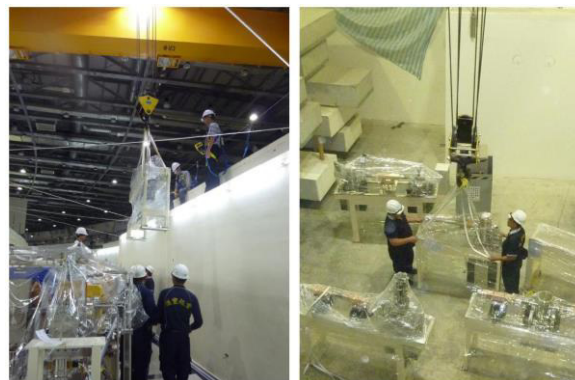
Figure 1: Transporting TPS front end subsystem table into tunnel.
