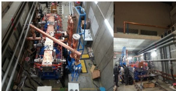
Figure 8: The connection from the amplifier to the cavity (two coupler ports).
