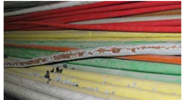
SPS irradiated cables Courtesy: D. Ricci
