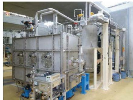
Figure 2: Installation of completed cERL injector cryomodule on beam line at injector section.
