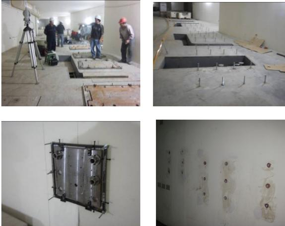
Figure 5: The construction of screw holes and bolt
