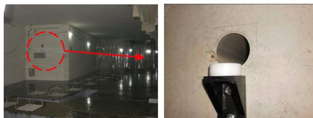
Figure 1: The storage ring and survey holes
