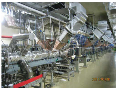
Figure 1: 100-MeV proton linac installed in the accelerator tunnel.
