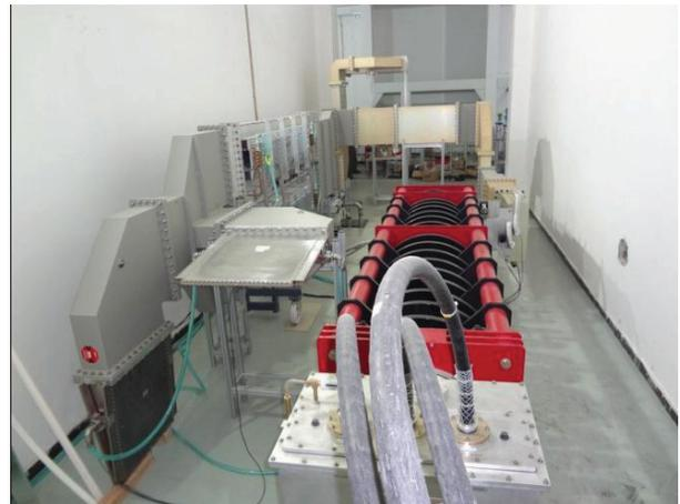
Figure 4: RF power system of CPHS linac
