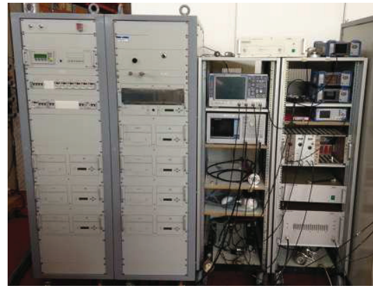
Figure 5: Power supply and measurement devices.
