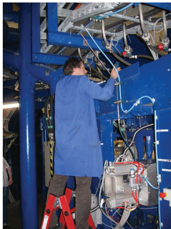
Figure 3: Inspection of water flow control units and thermo switches belonging to quadrupoles on the HIT ion gantry.
