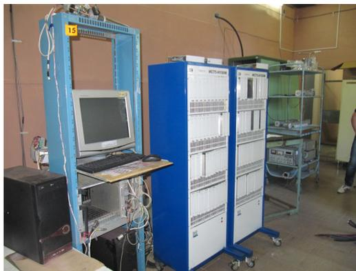
Figure 4: NESTOR facility storage ring magnetic elements power supply control system.
