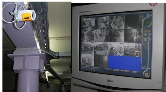
Figure 6: Elements of video monitoring system.
