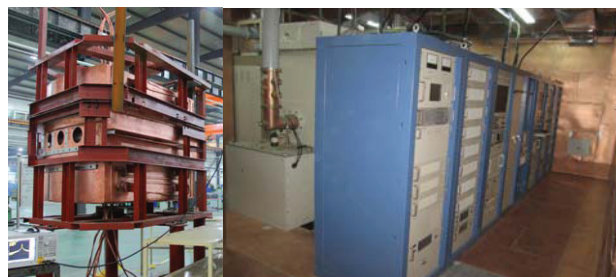
Figure 5: RF cavity (left) and RF power system in the shielding room (right).
