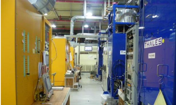
Figure 2: Three 300kW klystrons and KSUs.
