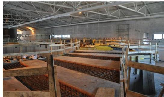
Figure 1: The roof of the storage ring tunnel.
