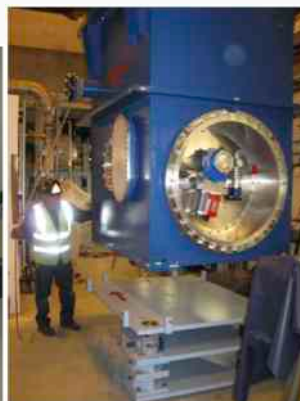
SRF gun In cryomodule
