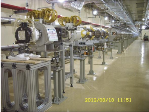
Figure 7: The installed 100-MeV linac in the accelerator tunnel at Gyeongju project site.
