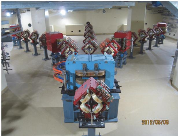
Figure 8: The installed 20-MeV beam line magnets in the 20-MeV beam line hall at Gyeongju project site.
