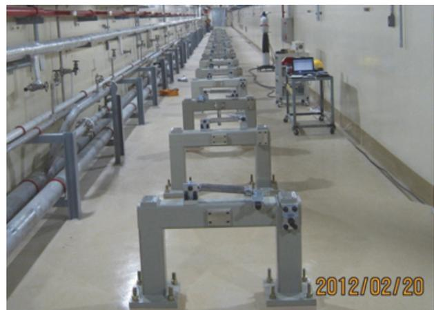
Figure 6: The linac supporting structure installed in the accelerator tunnel.
