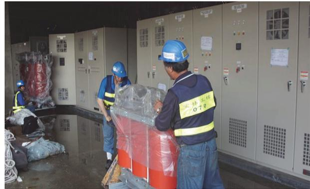
Figure 6: Installation of main electrical power equipment in one power substation.
