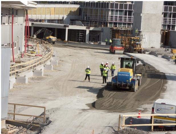
Figure 1: Installation of roll concrete for low vibration floor of synchrotron radiation beamlines end-stations.
