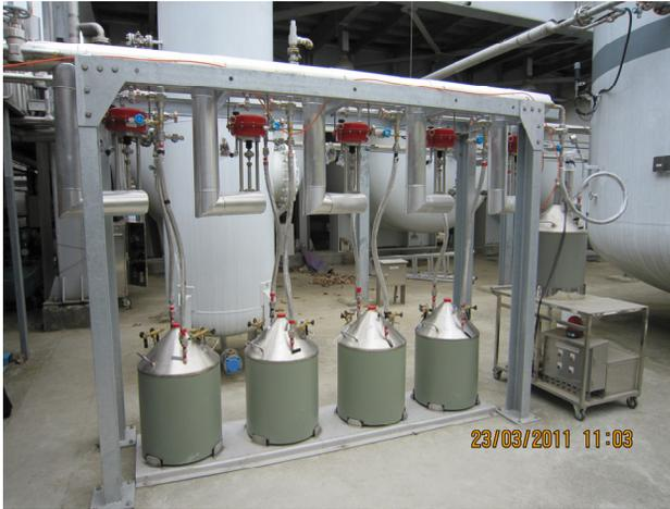
Figure 3: Adsorbers of the purifier system.
