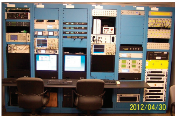
Figure 5: SRF Facilities Control Room.
