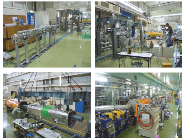
Figure 1: Status of construction and installation in Quantum Beam Project.
