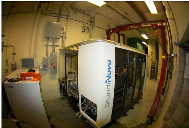
Figure 5: ScandiNova solid-state modulator installed at LLNL.
