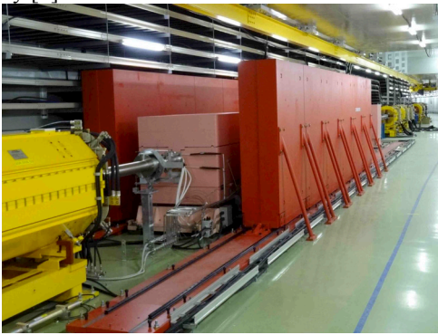
Figure 2; Iron shield walls installed in the MR collimator section.
