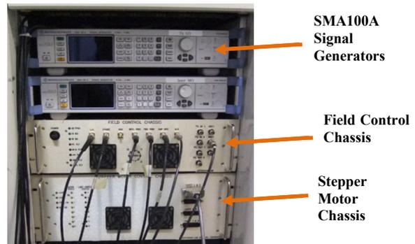
Figure 4: LLRF system installed in control rack.
