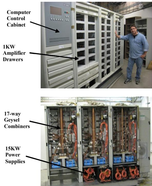
Figure 1: Front and back view of RF transmitter.
