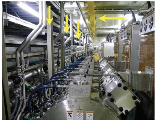
Figure 4: Separated cavity cooling system: Water Pipes are down from the ceiling (Flow rate: ~300 liters/min/station).
