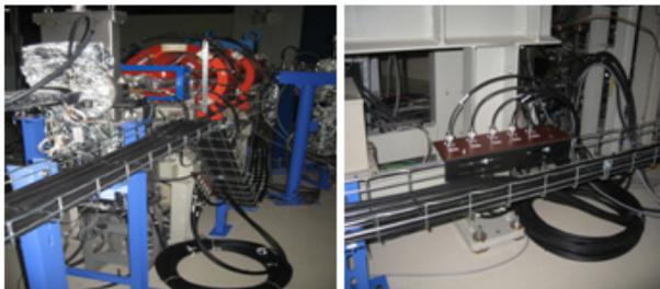
Figure 3: The new BPM signal cables installation.
