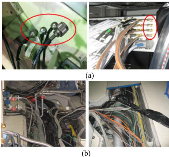
Figure 2: The original BPM cables and their installation.
