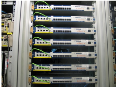
Figure 3: Seven Libera Single Pass installed.
