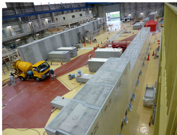
Figure 6: Installation of radiation shields for the cERL.
