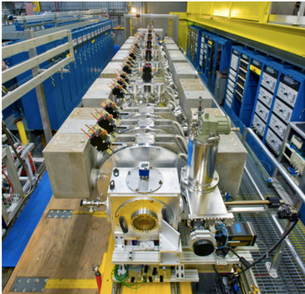
Figure 1: NDCX-II Facility. The injector is at the far end, with the diagnostic end station at the near end.
