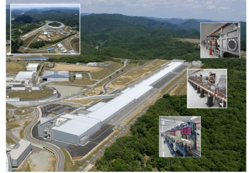
Figure 3: A bird eyes view of the SACLA facility. The electron beams are generated and accelerated from the right hand side to the left inside of the linac yard. The pictures of SPring-8 site and SACLA inside views are imposed.
