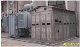
Figure 9: Choke and capacitor bank for White circuit of CSNS magnet power supply.
