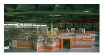
Figure 1: Photo of the radiation shielding wall in the center of experimental room (under-construction).
