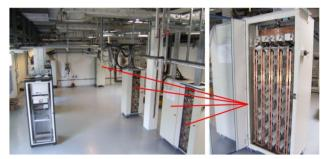
Figure 6: Booster transmitter room SYRF ready to receive 4 SSA (right: one 0.8 F capacitor bank for each SSA).
