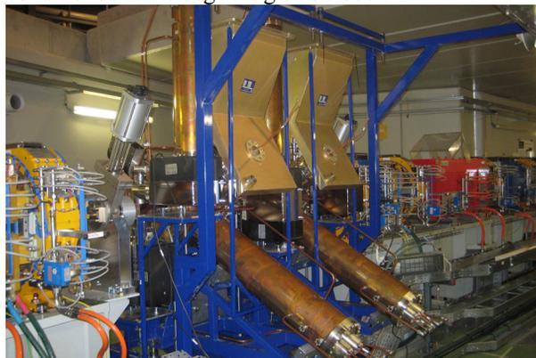
Figure 3: 2 Dampy cavities installed in one of the medium straight sections of the Storage Ring.
