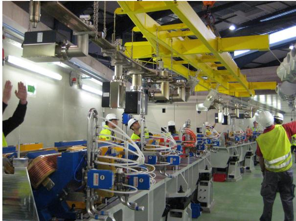
Figure 2: Installation of the vacuum chamber.
