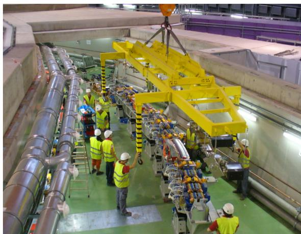
Figure 4: Installation of the vacuum chamber.
