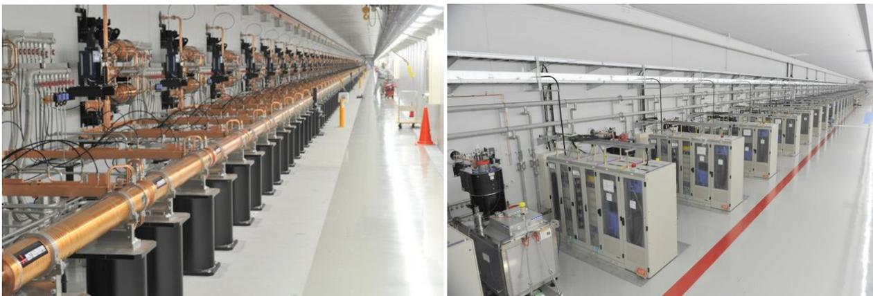
Figure 5: Left, C-band main accelerator in 400 m long tunnel; Right, klystron gallery. Compact modulators and controls.
