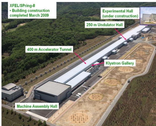
Figure 1: XFEL/SPRING-8 is under construction at SPRING-8 site.
