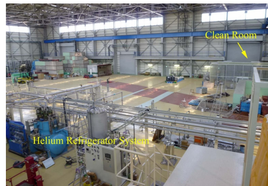
Figure 4: East Counter Hall after the refurbishment.
