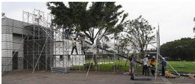
Figure 4: Scaffold to raise the flexible transfer lines from the grass yard to the TLS booster roof.
