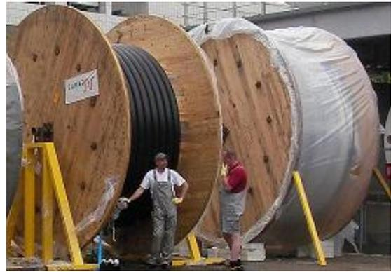
Figure 3: Flexible transfer lines delivered to NSRRC and the supporting frame to unroll these lines.
